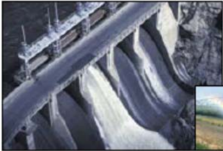
Flood Gate Control/Irrigation
